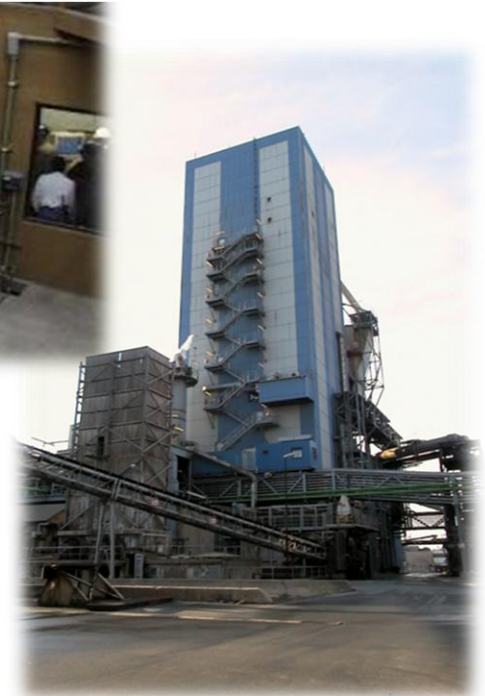
Lead Battery Recycling Recylex TSL (Germany)
